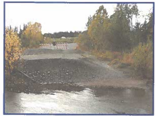
Restoration site - washout area and bank trampling from viewing and fishing. September 2006
