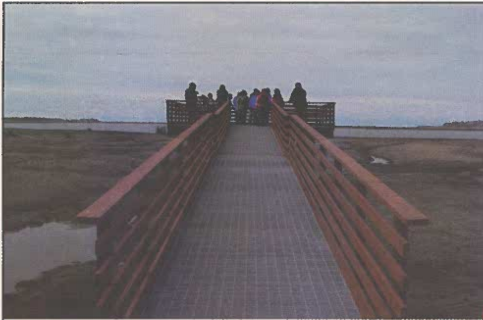
Wildlife and bird viewing platform near the mouth of the Kenai River.
