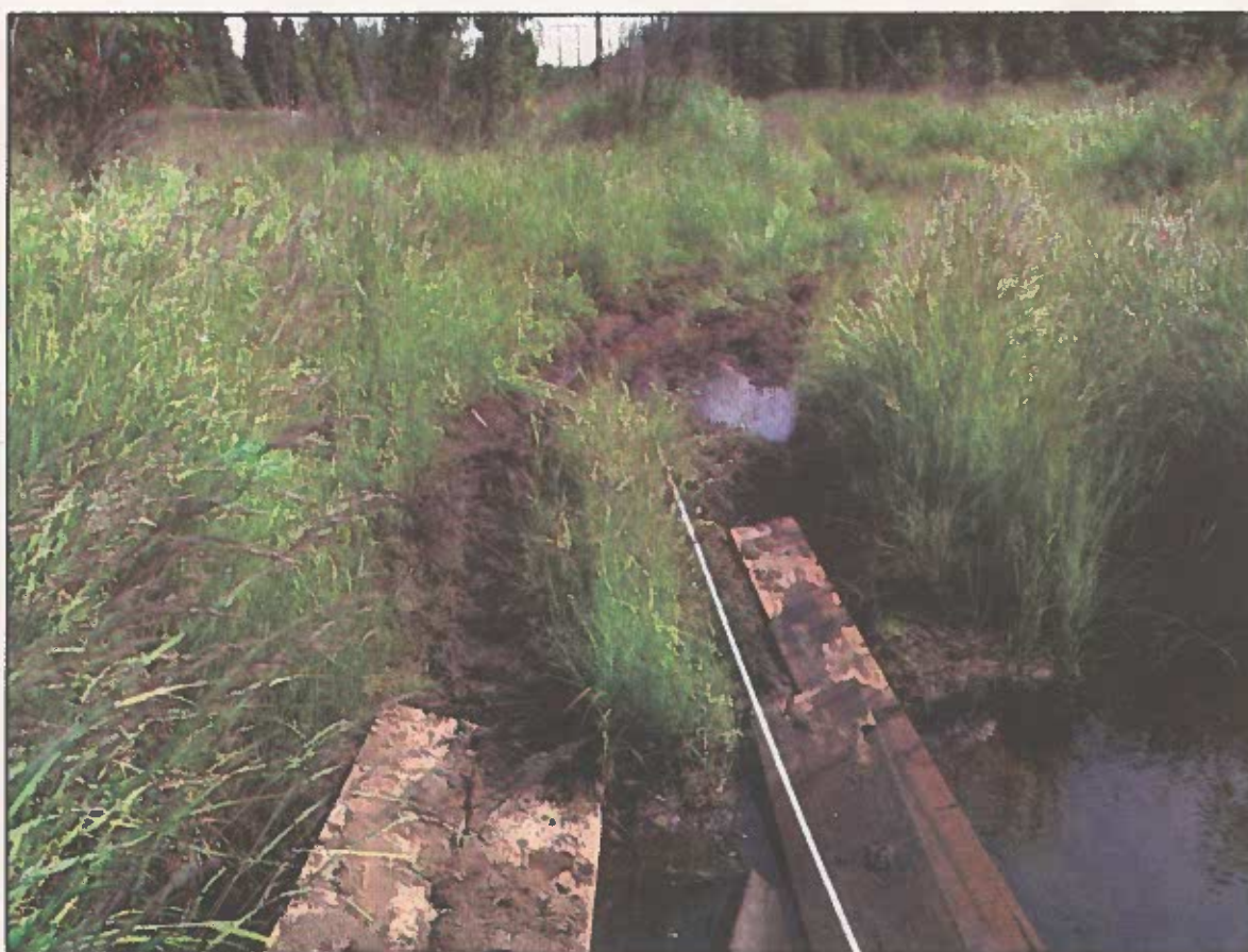
Unstable exposed sediment where a frequently used ATV trail crosses a wetland and salmon stream corridor.
