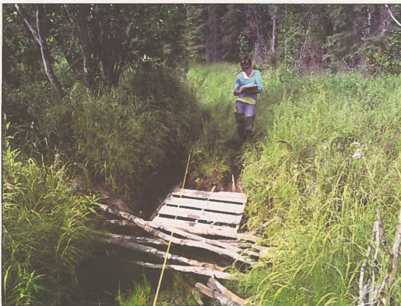
The pallet and logs used at another crossing site likely help to reduce sediment erosion into the stream, but they also might negatively affect salmon passage.
