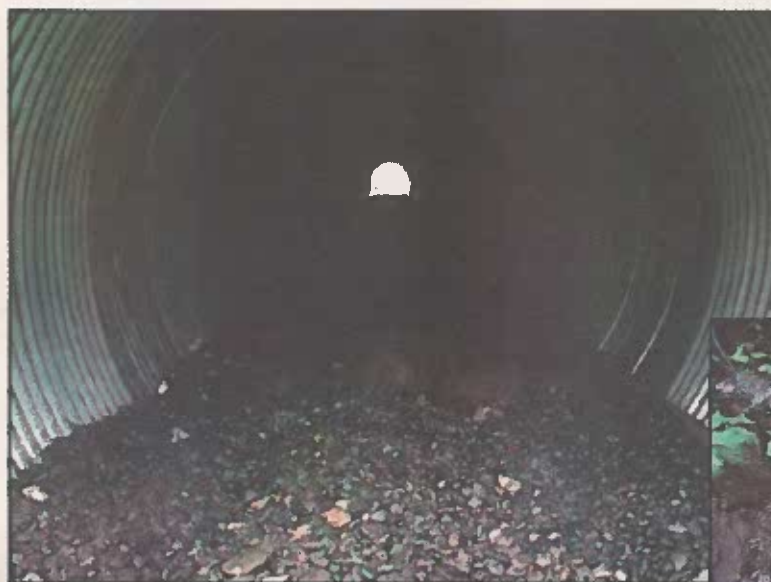
Photos: Above: Streambed installed. Right: Hydrolab monitoring of creek.
