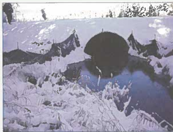
Far left: Culvert looking upstream before restoration
