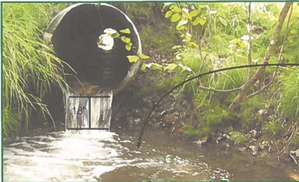
Culvert at Raven Road crossing of Bean Creek. This culvert was improperly sized and perched 18" above the stream. Juvenile fish cannot make this leap, so several miles of salmon habitat were blocked.
