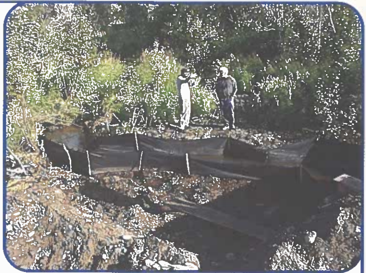
Above: Construction and restoration underway.
