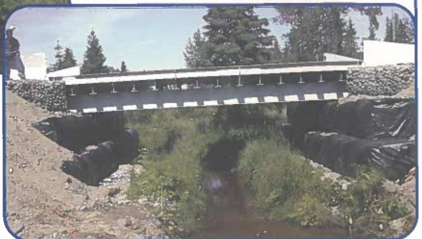
Henry's Creek - The bridge spans the channel and a significant portion of the floodplain. Wider span bridges more closely mimic the natural conditions of streams and are beneficial to fish and all aquatic life.
