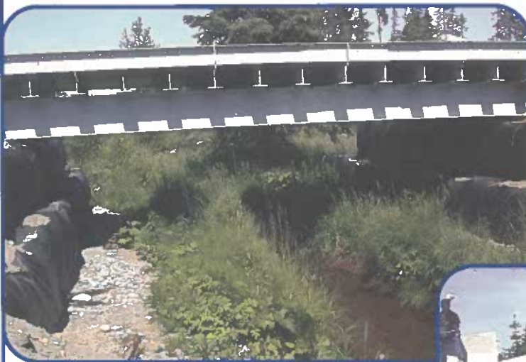
Henry's Creek - The bridge spans the channel and a significant portion of the floodplain. Wider span bridges more closely mimic the natural conditions of streams and are beneficial to fish and all aquatic life.
