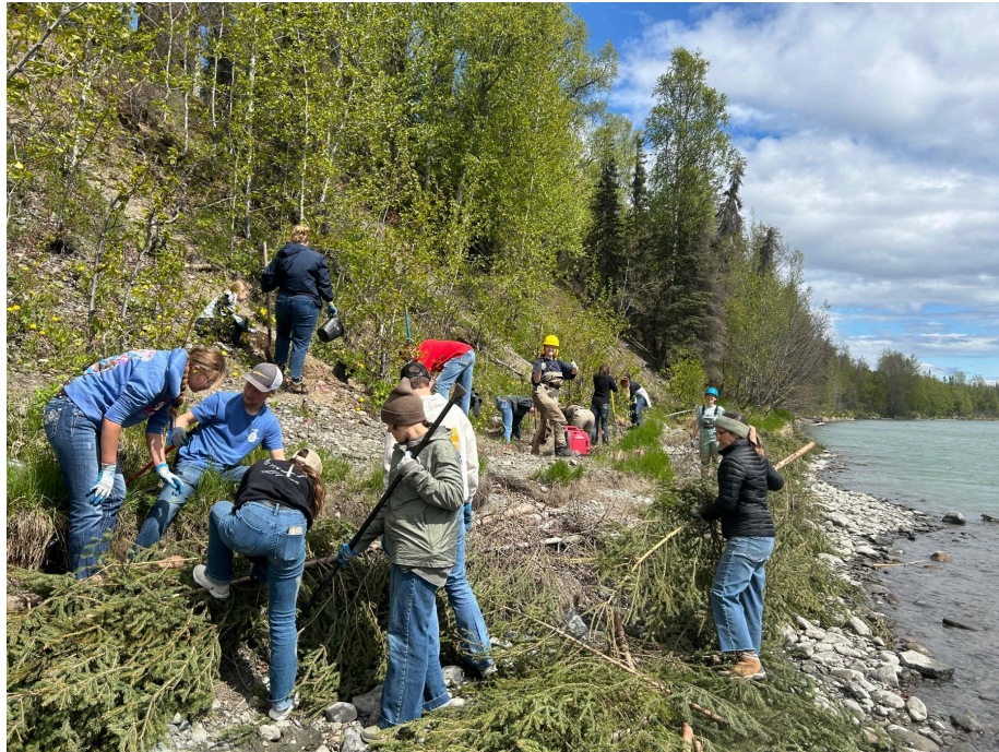
FFA group performing spruce tree cabling and revegetation along the Kenai River. (Drzazgowski, 2024)
