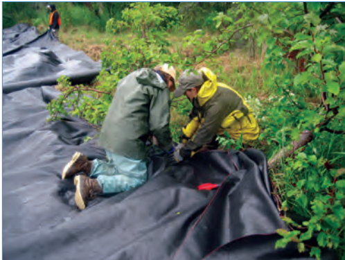
Left: Stephanie and Jan install typar around a tree at Beaver Creek
