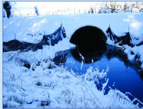
Far left: Culvert looking upstream before restoration
